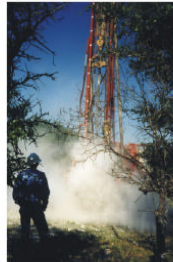
An air rotary drill rig was brought in to drill at the location of the suspected cave. When the rotating hammer bit hit the "cave", a huge cloud of dust was brought up to the surface. The suspected cave turned out to be a gypsum bed.
