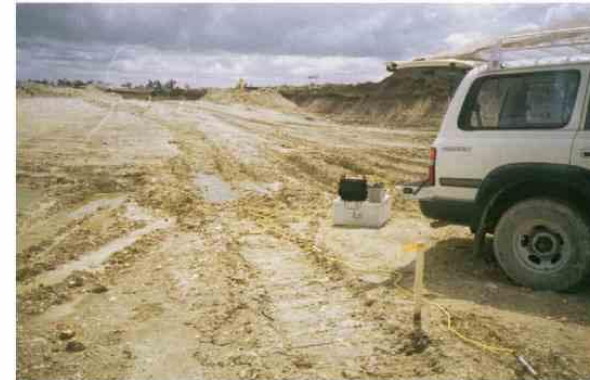
The survey site after 3 meter of conductive top soil had been removed.
