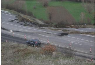
Our client, the Geophysical Modeling Group from Ankara University, Turkey, used AGI tools to investigate the landslide's bedrock and weak zone. The goal of this study was to delineate the landslide's body and slip plane depth and take measurements before reconstructing the highway.
