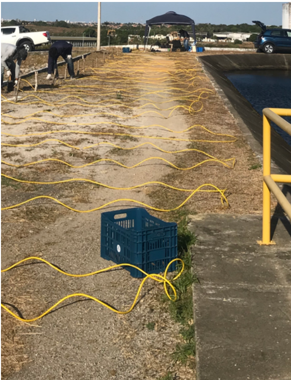
Pictured above: The placement of the 37 electrodes installed on the dam's crest. The space between each electrode was 2m.
