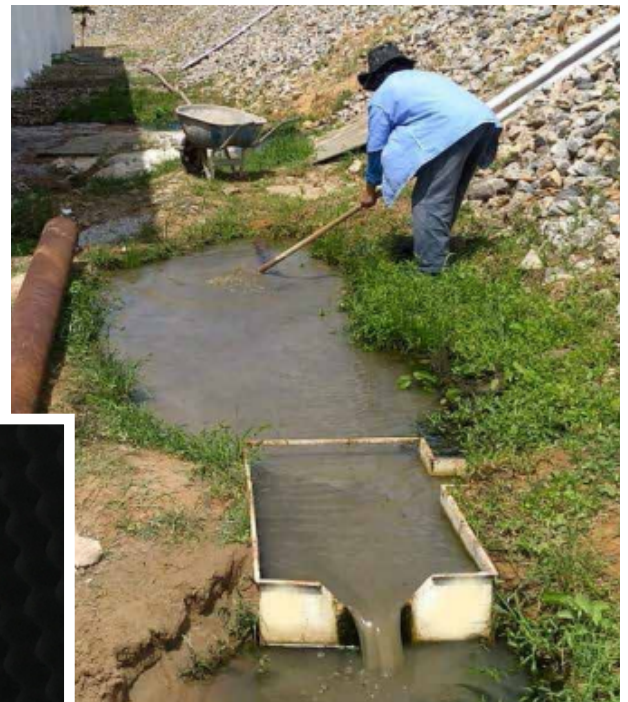
Pictured above: Visible surface leakage from the dam.
