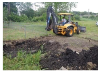
Excavation of 3D resistivity anomaly
