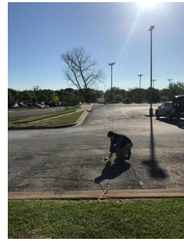
Installation of passive cable for ERI survey
