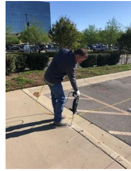
Drilling of asphalt/concrete for electrode stake installation
