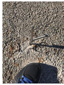
Installing electrode stake in asphalt/concrete for ERI survey
